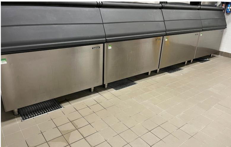
Stainless steel box channels with mesh gratings in the area of ice cube machines.
