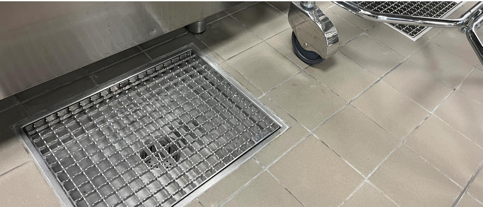
Waters in all professional kitchens are collected and treated with high quality stainless steel drainage and grease separation systems from ACO
