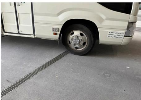
Line drainage with stainless steel gratings on delivery entrance ramp
