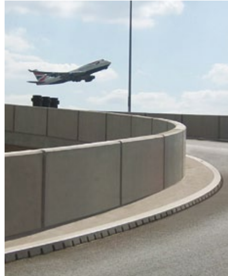
Shallow depth ACO KerbDrain installed along vehicle entry and exit ramps of multi-storey car park
