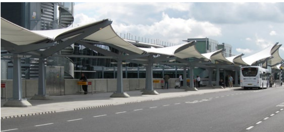
ACO KerbDrain used to drain surface water from the new passenger set down area
