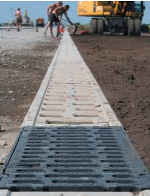
Drainage channel / inlet box
