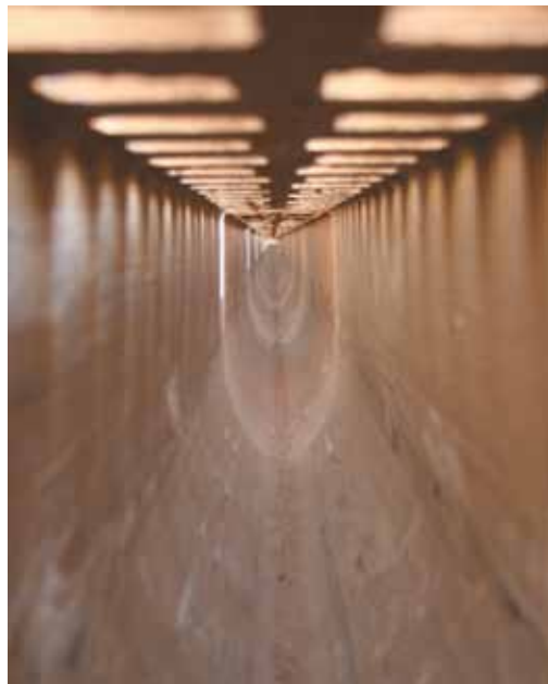
Look at the miles of extensive drainage line
