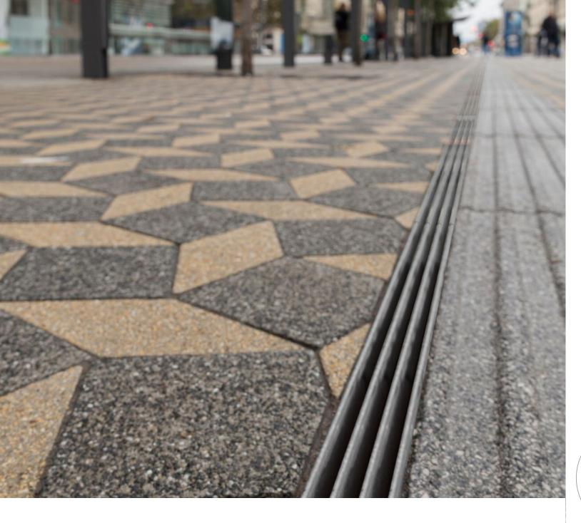
SlotTop Triple is the playful variant. In combination with a colourful or patterned paving it creates a exciting design. It highlights drainage and enables architects to underline, how functional elements can become aesthetical details. As an additional quality, the SlotTop Triple has an even bigger intake area.
