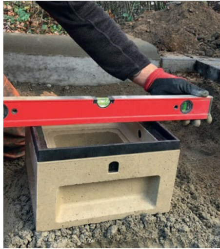
Alignment of the drain body in the concrete bedding
