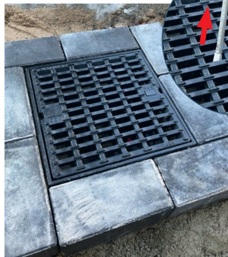
Insertion of the cover grating. The grate is secured after the lock engages.
