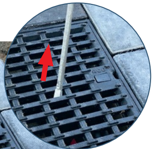
Jerky lifting of cover grid with the help of grating hooks
