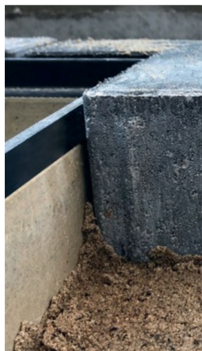
Built-in 3-5mm raised Plaster around the drain body
