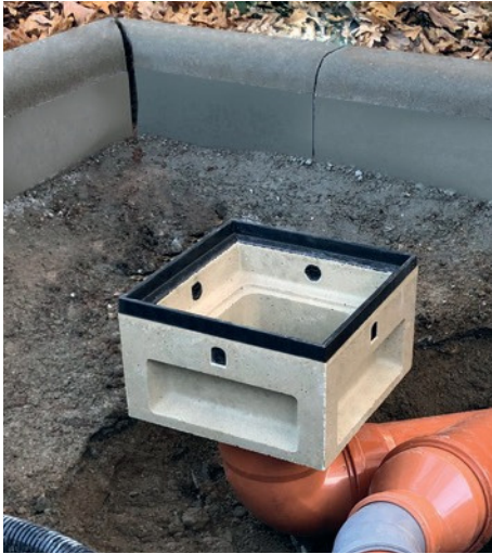
Multipoint D 400 with a cast frame in the short version
