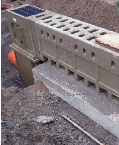
ACO DRAIN® Monoblock RD 300 DF on the A3 motorway at Cologne
