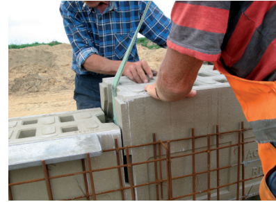
Laying ACO DRAIN® Monoblock RD 300 D
