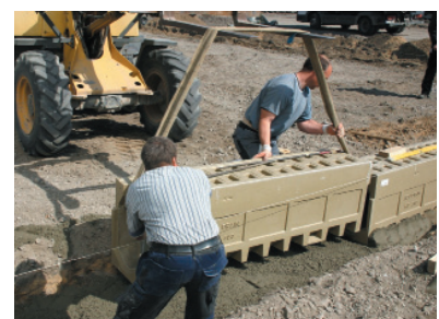
ACO DRAIN® Monoblock RD 300 being installed
