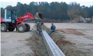
ACO DRAIN® Monoblock RD 300 DF at an airport
