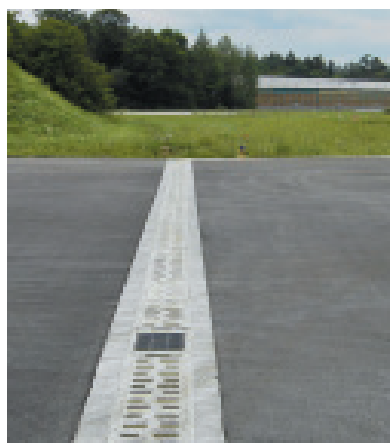
ACO DRAIN® Monoblock RD 300 at Manching airport with outlet shaft
