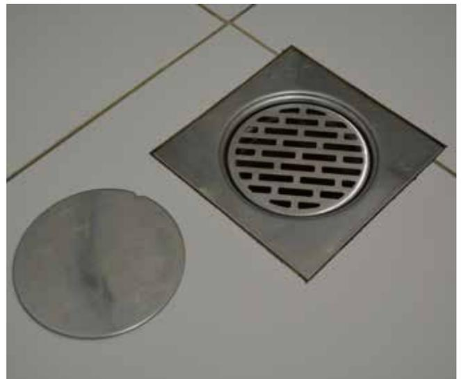
**ACO Floor Drains as standard floor drainage solution**
