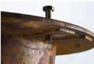
Because the bolt goes right through the flange, long-term safe sealing is impossible.
