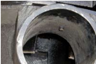
A drain with screws in the piping means complete sealing is impossible.
